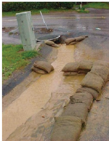
Figure 5. Make sure storm drain inlets are protected.
